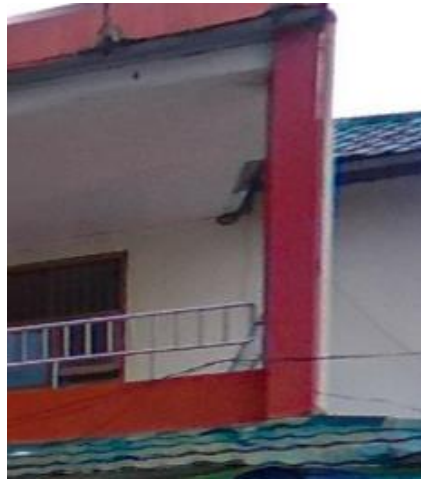
Figure 2. 3 Building Equipped with Standpipe
