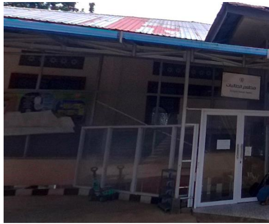
Figure 2. 2 Building Equipped with Gutter
