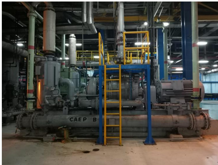
Gambar 5.46 Condensate Air Extraction Pump
