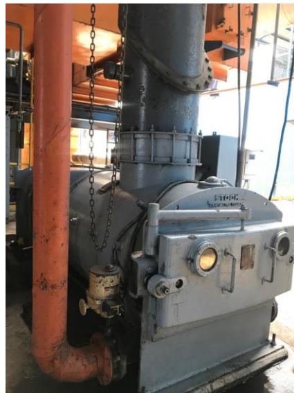
Gambar 5.29 Coal Feeder
