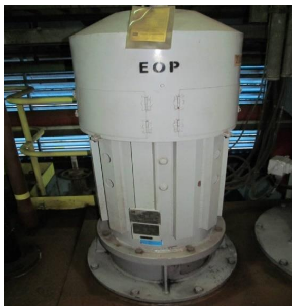
Gambar 5.52 Emergency Oil Pump
