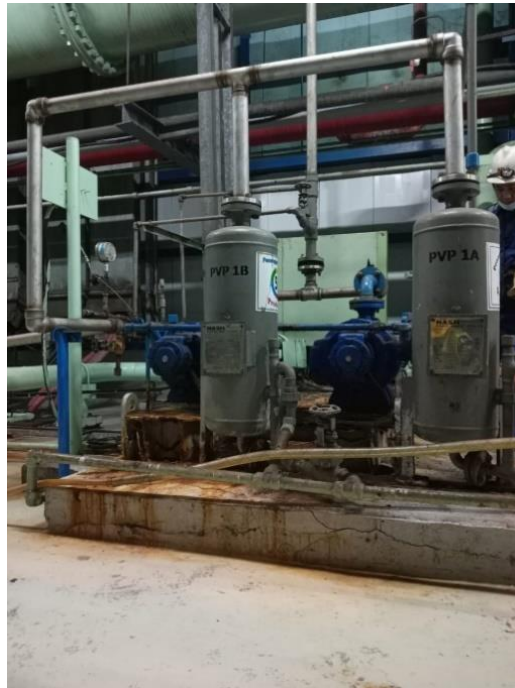
Gambar 5.47 Priming Vacuum Pump
