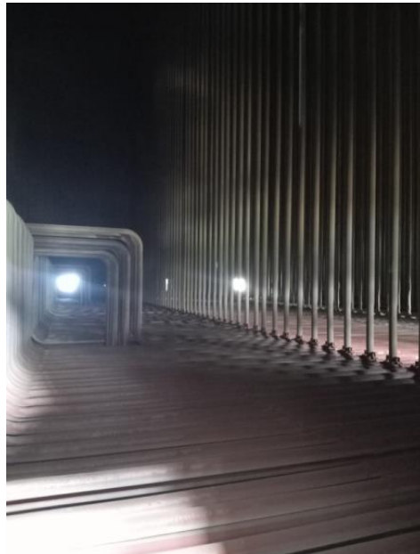
Gambar 5.13 Superheater
