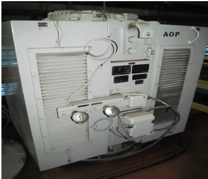
Gambar 5.54 Auxiliary Oil Pump
