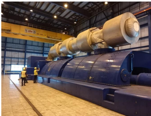
Gambar 5.15 Steam Turbin
