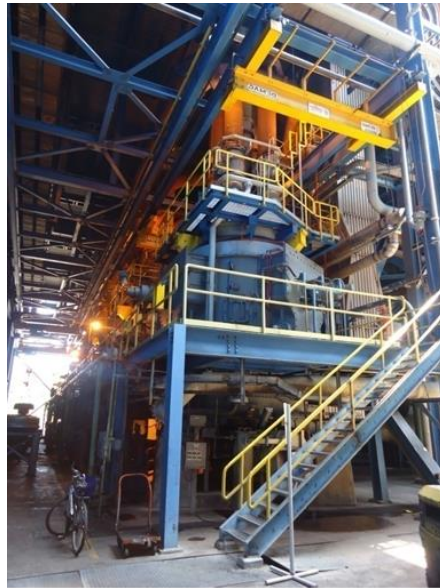
Gambar 5.30 Pulverizer
