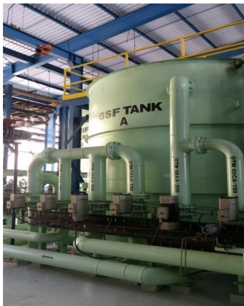
Gambar 5.58 Gravity Sand Filter
