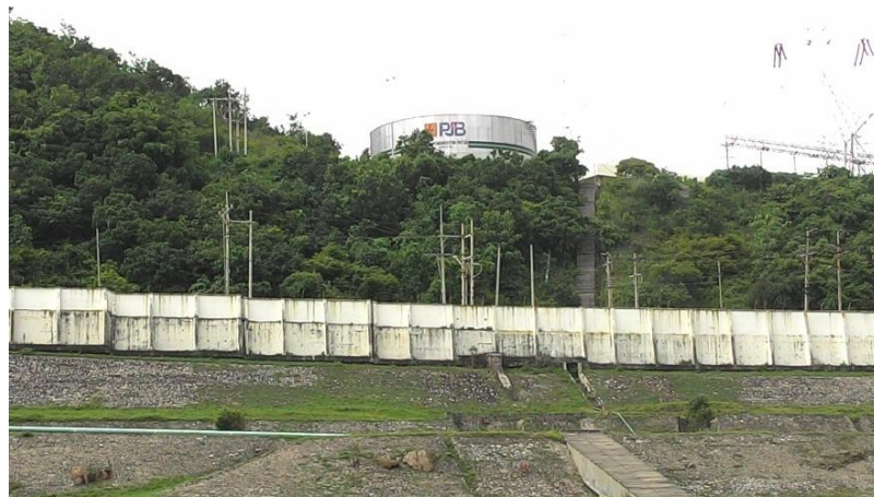
Gambar 5.56 Services Water Tank
