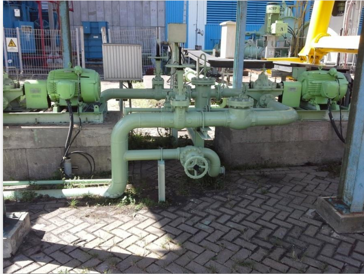
Gambar 5.49 Condensate Transfer Pump
