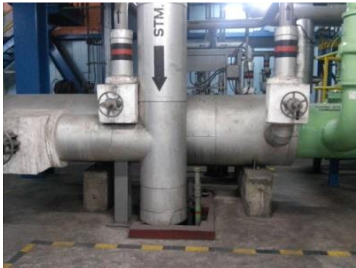
Gambar 5.50 Gland Seal Condenser
