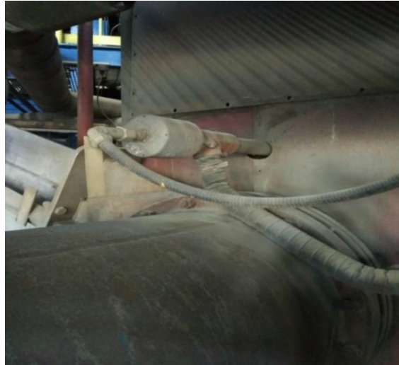
Gambar 5.41 Flame Scanner
