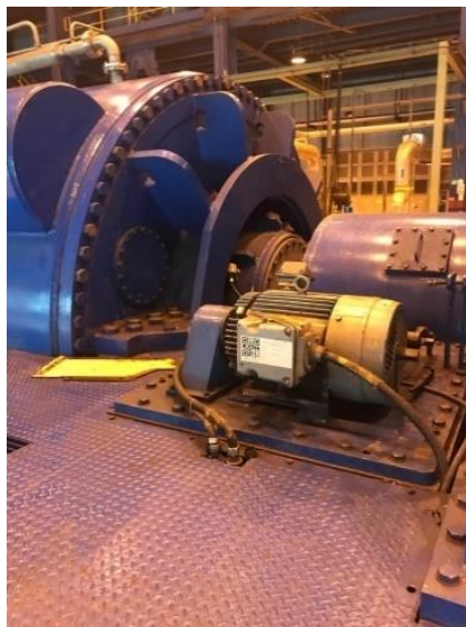
Gambar 5.17 Turning Gear Motor
