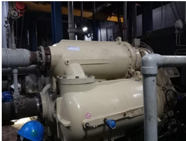
Gambar 5.42 Air Compressor
