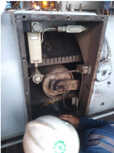
Pengecekan Belt Conveyor Coal Feeder
