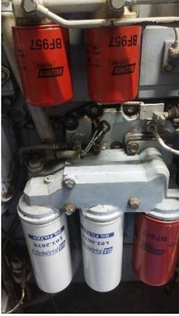
A close-up photograph of the maintenance area of a generator set. It shows several cylindrical filters: two red ones at the top with 'BF957' printed on them, and two white ones below with 'MANN-ESB' branding. A red filter is also visible on the right side. |
