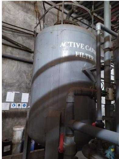
**Gambar 4.27** *Active carbon filter* di *power house*
