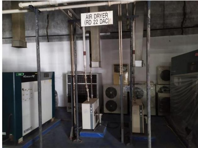
**Gambar 4.8** *Refrigated Air Dryer di power house*
