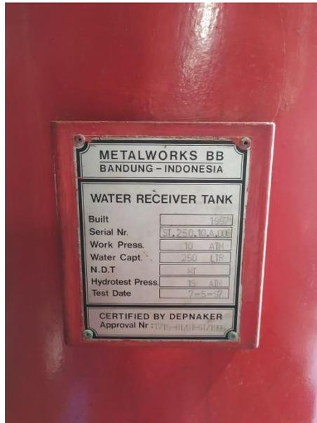
**Gambar 4.21** Spesifikasi *Water Reciever Tank Hydrant Pump* di *Power House*
