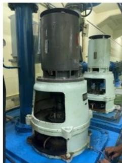
Gambar 4.4.2 1 Tampak Motor Pompa Centrifugal Drainage Pump
