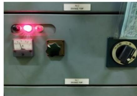
**Gambar 4.3.2.2 Activation Indicator at MCC for pump no, 1 (Active)**
