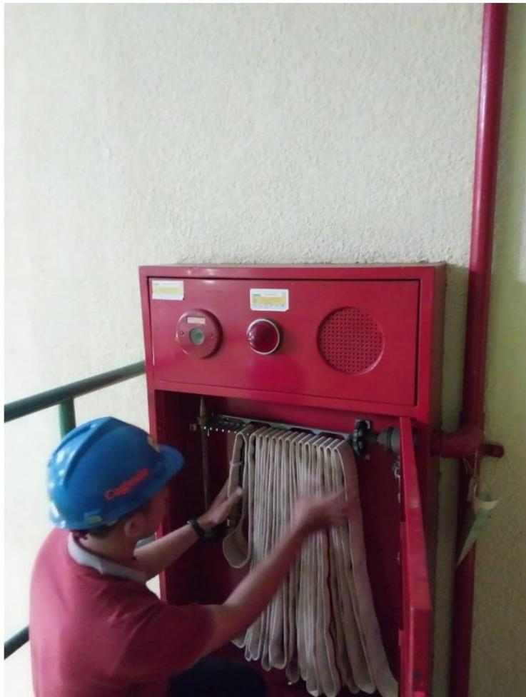
Gambar 4.2. 5 Pengecekan APAR & Hydrant
