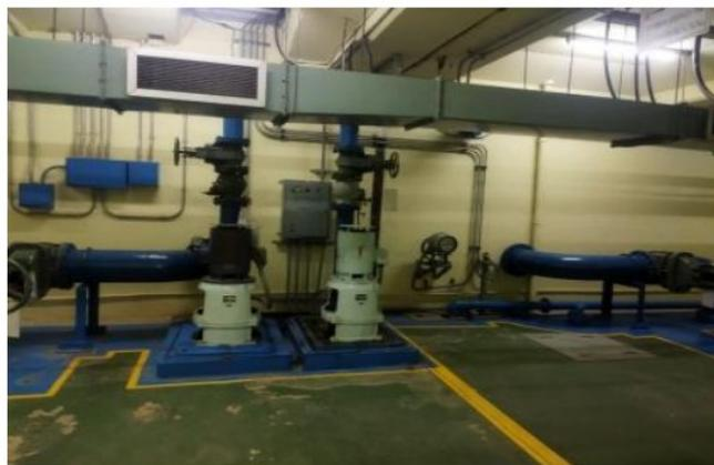
Gambar 4.3. 1 Drainage Pump
