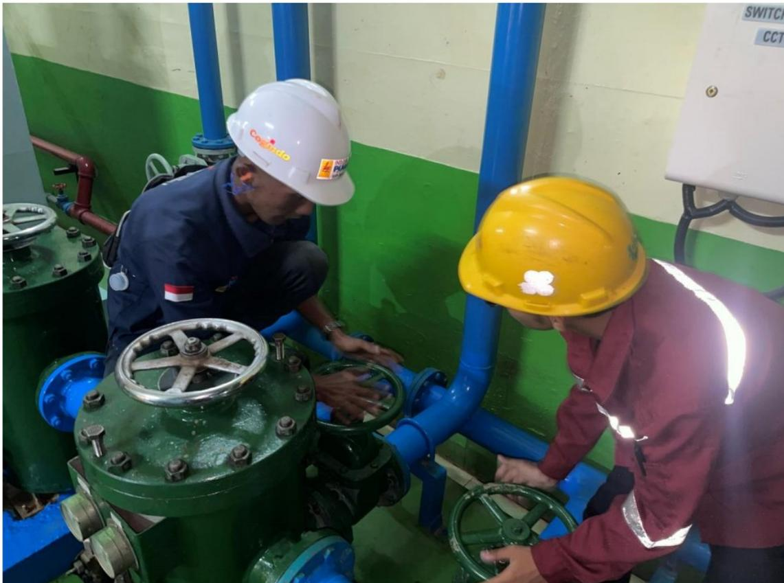
Gambar 4.2. 4 Perawatan Cooling Water Strainer
