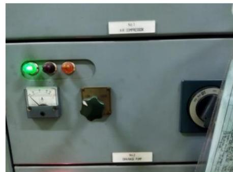
**Gambar 4.3.2.3 Activation Indicator at MCC fot pump no. 2 (Deactivated)**
