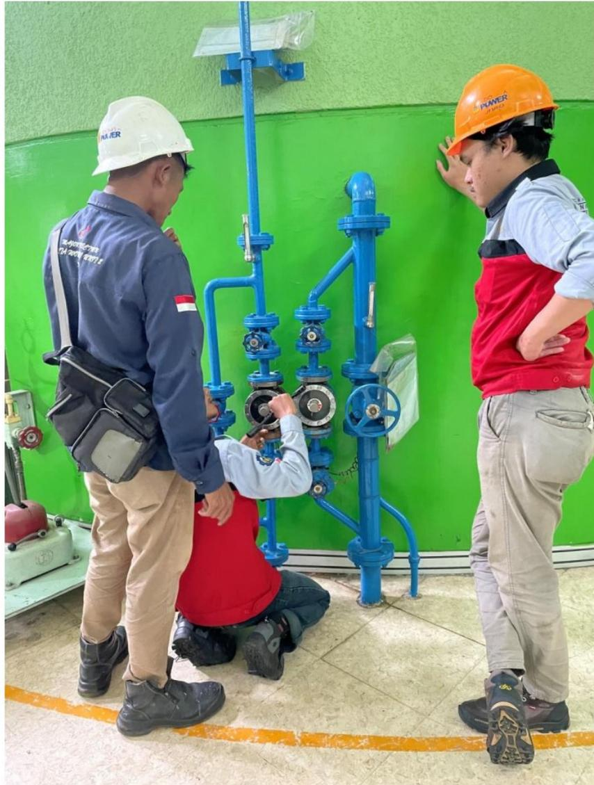
Gambar 4.2. 9 Pengecekan Bearing Cooler Waterflow Indicator
