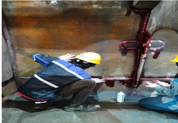
**Gambar 4. 9** Proses Pemberian Liquid Penetrant
