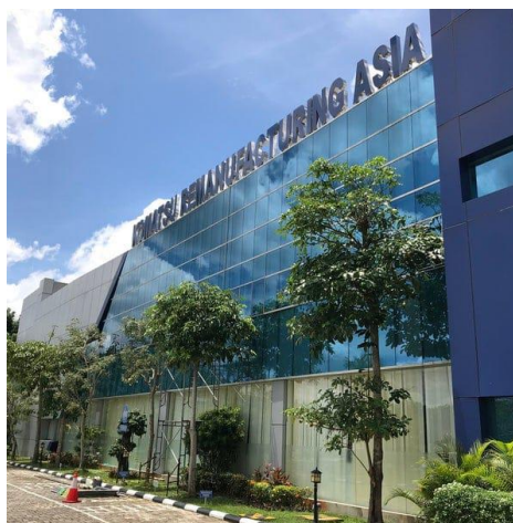
Gambar 2.5 Plant Balikpapan PT Komatsu Remanufacturing Asia (Sumber : PT. Komatsu Remanufacturing Asia)
