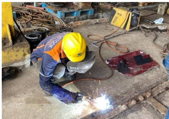
**Gambar 3.20** Mengelas *Mounting Jembatan (Apron)*
