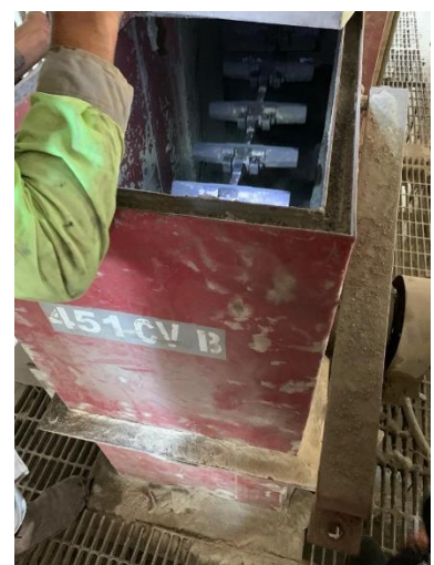
Inspection 451 CV B
