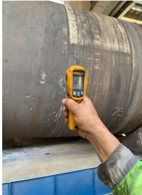
Inspection Kiln Tuban 1
