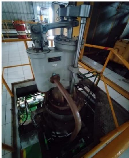
**Gambar 2.3** Main Stop Valve Turbin Uap Unit 1 PLTU Jeranjang OMU
