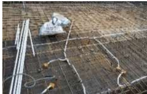
Gambar 6.18 Pemasangan Pipa Mechanical Electrical
