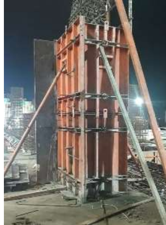
Gambar 4.11 Pengecekan Verticality Bekisting Kolom dan Shear Wall
