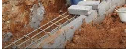
Gambar 4. 12 Pekerjaan Bekisting Tie Beam
