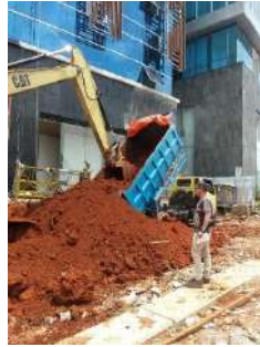
Gambar 4. 8 Pekerjaan Urugan Tanah(Sumber : https://jasaurugtanah.com/blog/category/urugan-tanah-merah )
