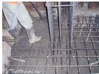
Gambar 4. 11 Proses Perataan Beton Pilecap
