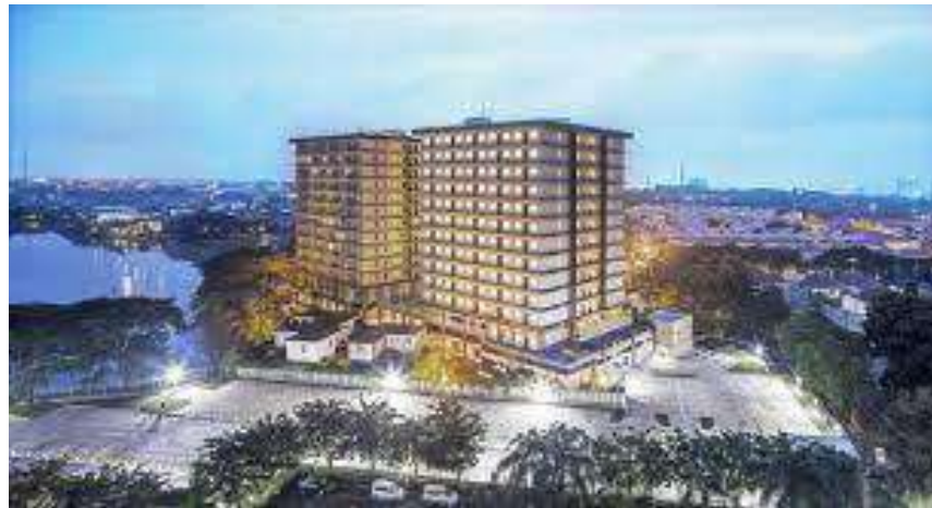
Gambar 1. 3 Gedung Hotel Axia South Cikarang Sumber: Google Image
