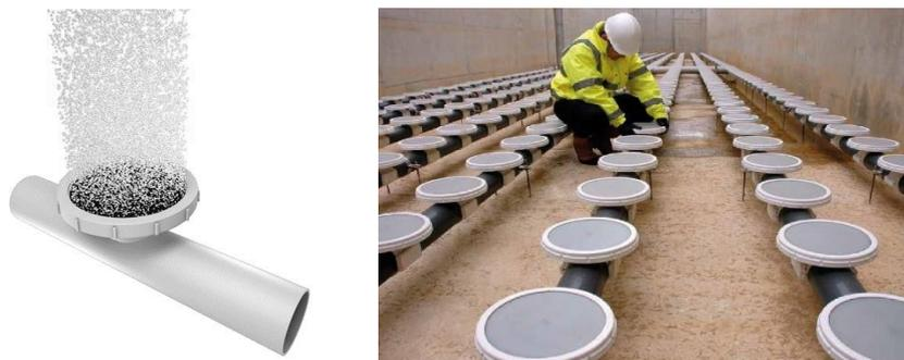
Gambar 2.5 *Disc Diffuser*
