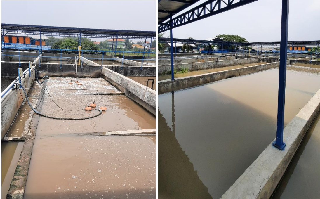
Gambar Unit Prasedimentasi IPA Siwalanpanji
