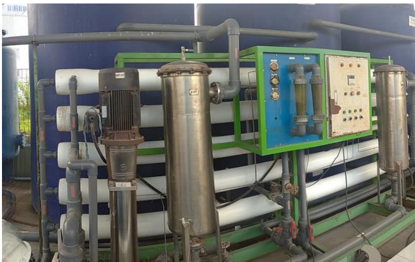
Unit Nanofilter IPL TPA Benowo
