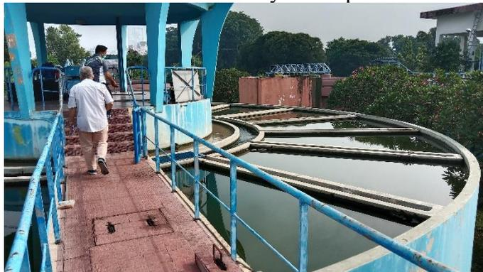
Gambar 3.3 Unit *Accelerator* IPAM PDAM Ngagel II
