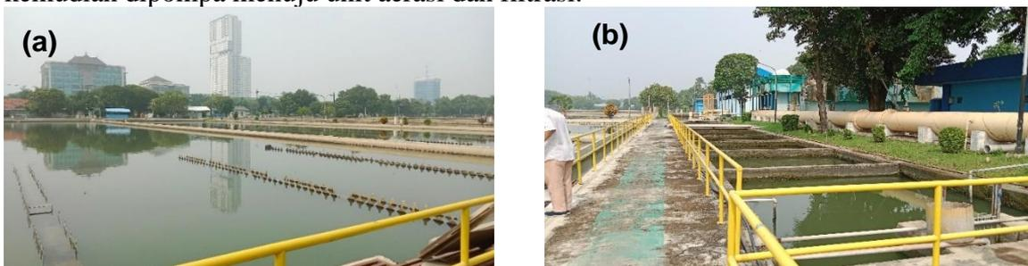
Gambar 2.2 (a) Unit Sedimentasi IPAM PDAM Ngagel III Surabaya, (b) Kanal III
