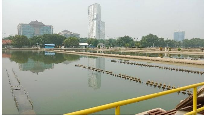
Gambar 3.4 Unit Sedimentasi IPAM PDAM Ngagel III
