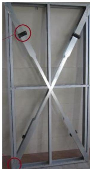
Gambar 2.6 *Conventional construction CFS light-frame strap braced wall systems*
