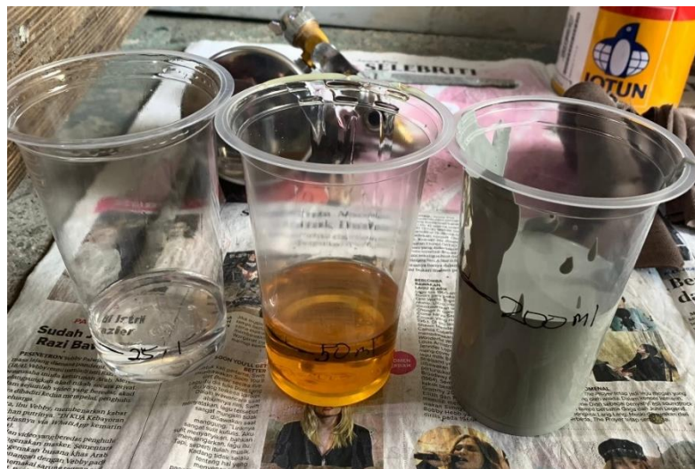
Gambar 3.17 Persiapan Campuran Cat Epoxy
