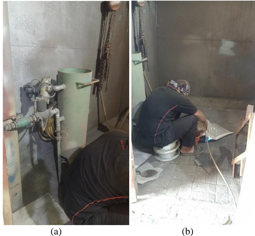
Gambar 3.11 (a) Alat Dry Abrasif Blasting , (b) Proses Blasting
