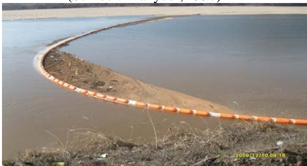
Gambar 5.30 Silt Barricade (Sumber: erosionpollution.com)
