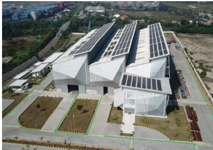
Gambar 12.1 PLTS Atap Workshop PT. Barata Indonesia
