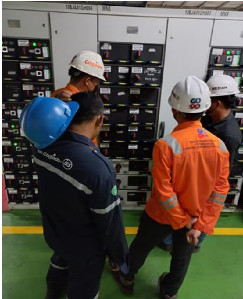
Gambar 4.4 Melaksanakan Rack-In Breaker 380 V.
