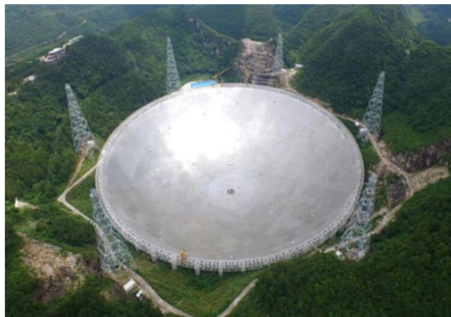
Figure 2.5 Application of CDPR in large spherical radio telescope (Duan et al., 1999)
