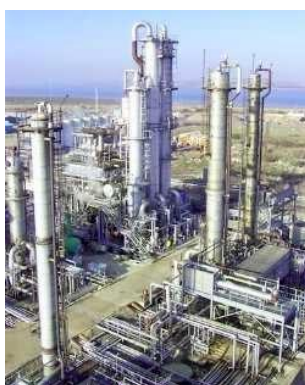
Gambar 2.7 Proses Separator Column Sumber : (Drieant, 2014)
