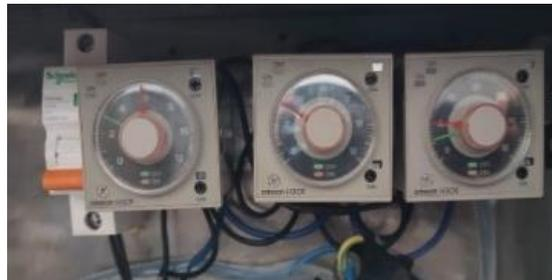
**Gambar 4. 25** Timer Delay Relay
