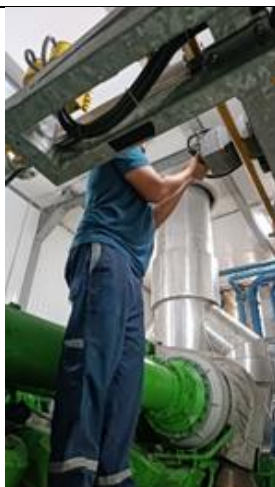
Melakukan pengecekan Throttle Valve dikarenakan gagal start engine
