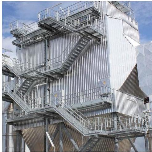
**Gambar 4.10** *Electrostatic Presipitator*
