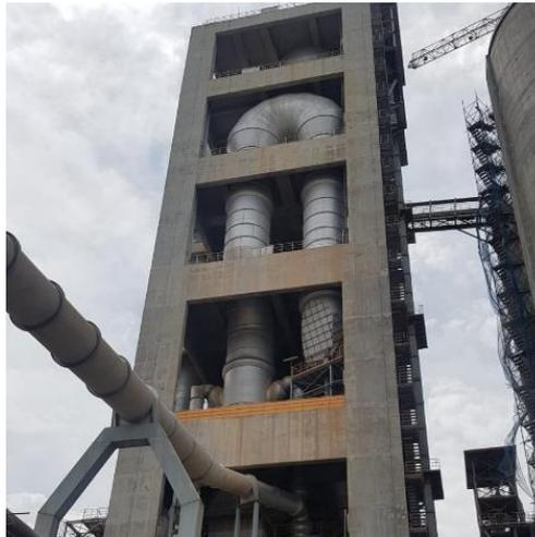
**Gambar 4.7** *Suspension Preheater*
