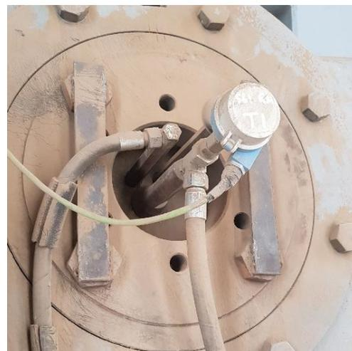
**Gambar 4.25** *Analog Temperature Sensor*
