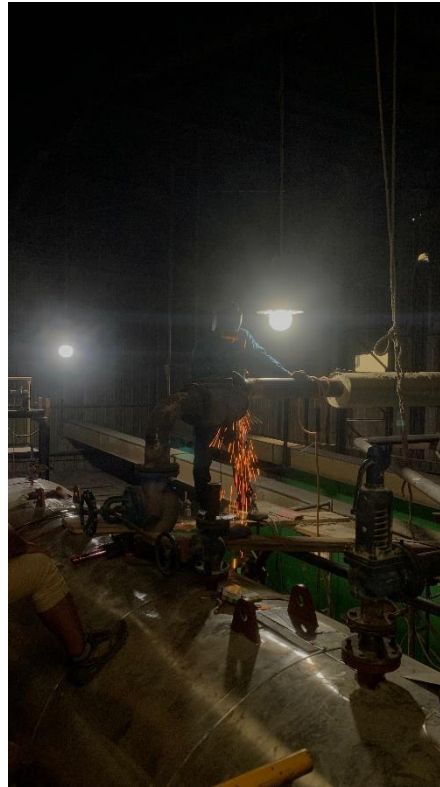
Gambar 4. 16 Pekerjaan Connecting Piping Main Steam Valve & All ACC (Sumber: Dokumentasi Pribadi)
