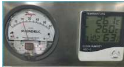
Gambar 4.19 Differential Pressure Room & Digital Thermo Hygro Sumber : Dokumen Pribadi PT Sampoerna Tritunggal Pratama
