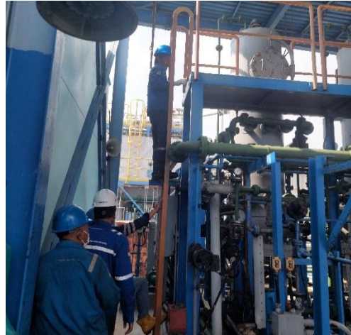
Gambar 4. 19 Area Water Treatment Plant
