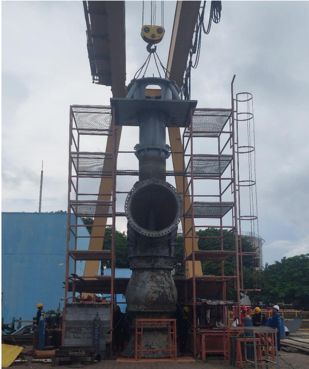
Gambar 4. 26 Circulating Water Pump
