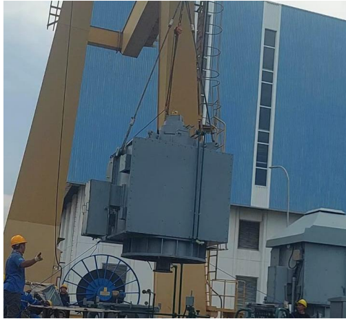
Gambar 4. 28 Motor Circulating Water Pump
