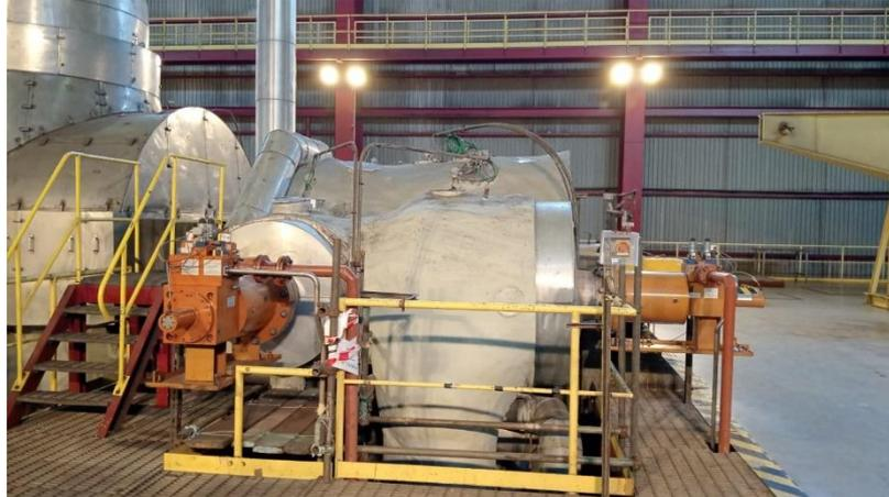
**Gambar 2. 9** *High Pressure Turbine*
