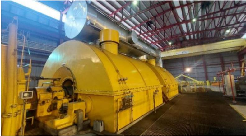
**Gambar 2. 11** *Low Pressure Turbine*
