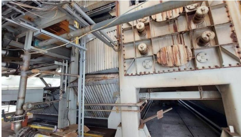
**Gambar 2. 37** GGH (*Gas-Gas Heater*)
