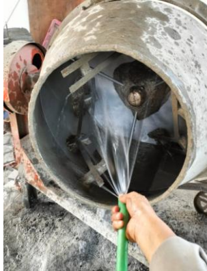
Gambar 3. 8 Pengondisian Alat Mixer Beton
