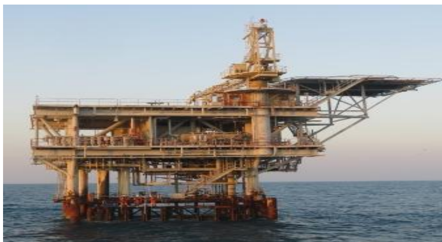
Gambar 4.2 Offshore Platform AAC-Well
