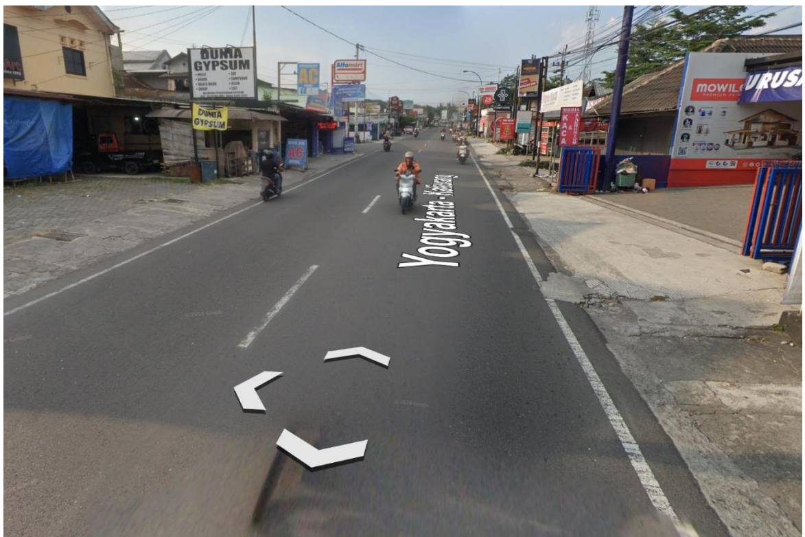
Gambar 5. 9 Gambar Lapangan STA 6-7 Yogyakarta-Kaliurang
