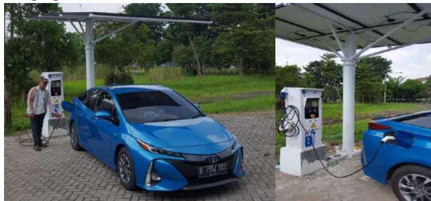
Gambar 2.32 PV Charging Station
