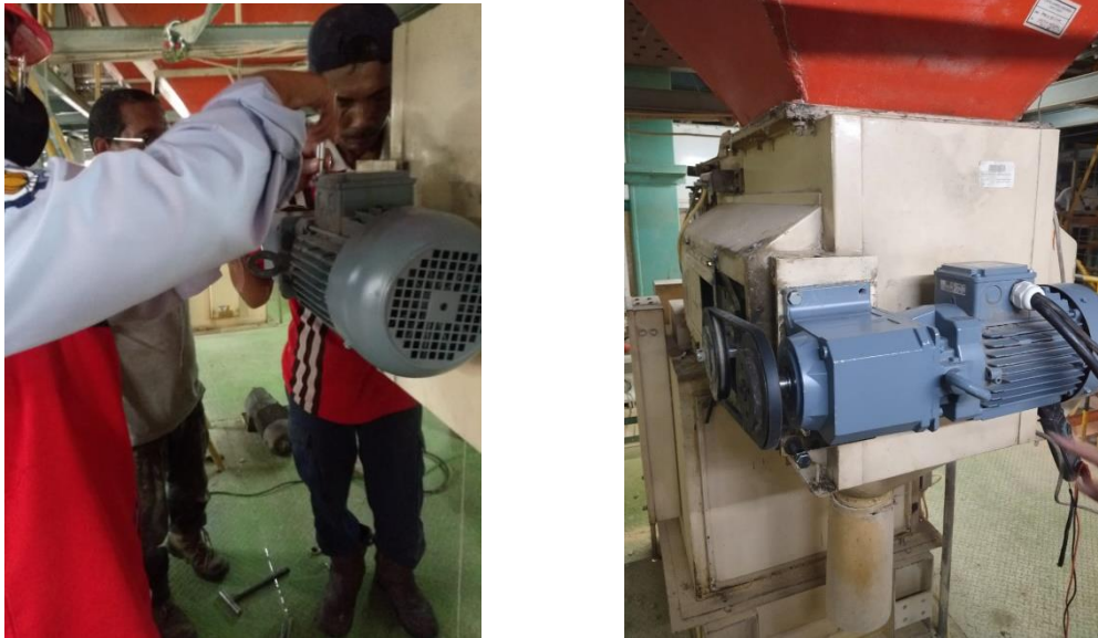
Gambar 3. 6 Maintenance Chronos Bagger
