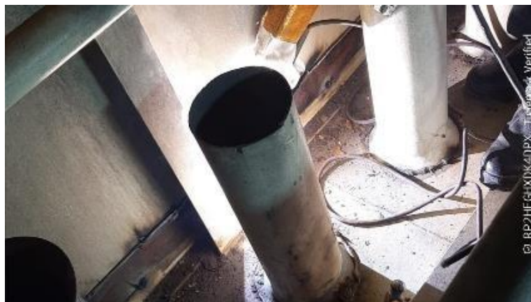
Gambar 4. 25 Repair Pipe Extension IAF
