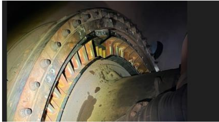
Gambar 4. 32 30 Pengecekan Kondisi Coating Turbin Blade no.1
