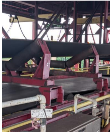
Gambar 4. 23 Belt Conveyor
