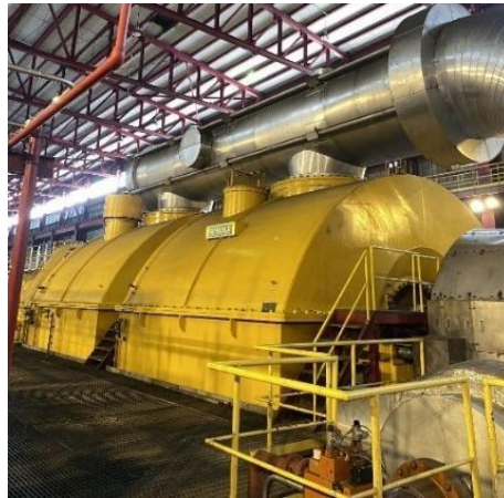
Gambar 4. 14 Intermediete Pressure Turbin
