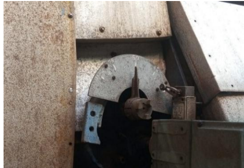
Gambar 4. 29 Blade Pitch Adjustment
