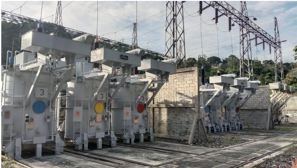
Gambar 4.17 Transformator
