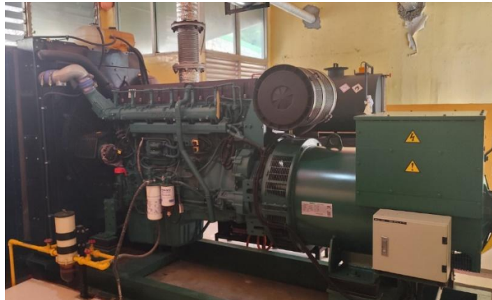
Gambar 4.12 Mesin Diesel Darurat ( Gen-Set )
