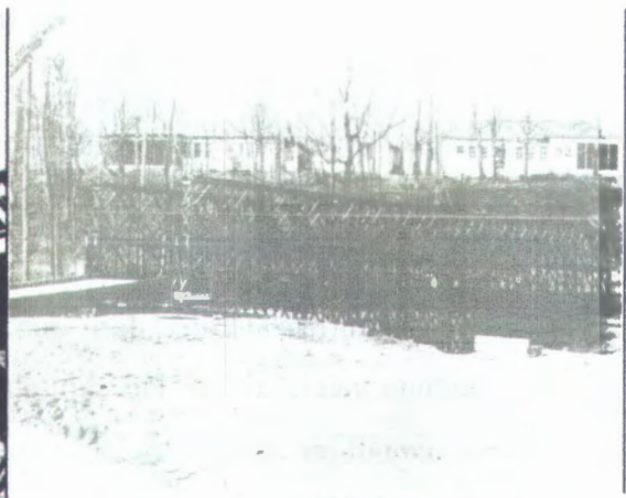
Figure 2-7. Double-double Bailey bridge.
