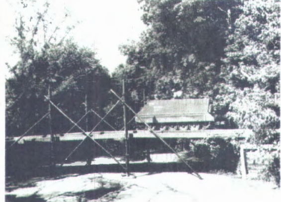
Figure 2-9. Class 60 M4 truss bridge, aluminum.
