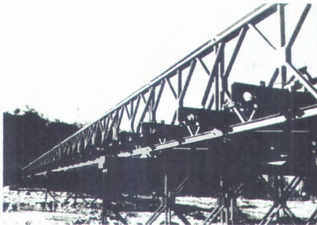
Figure 2-6. Bailey bridge using Bailey panel piers.
