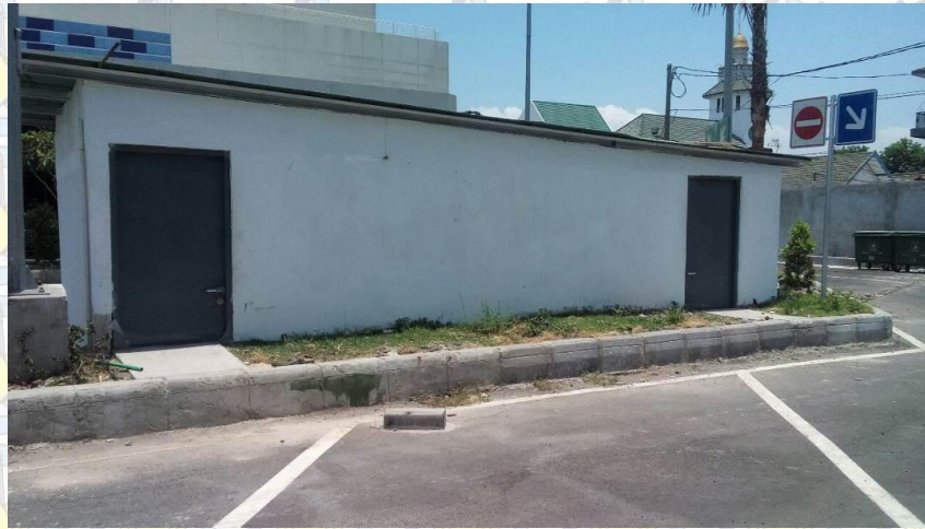
Gambar 4.22 Sewage Treatment Plant milik terminal GSN.
