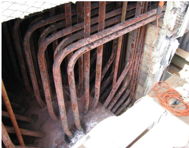
Gambar 2.6 Desain feedwater drum dan bend tube preheater [6]
