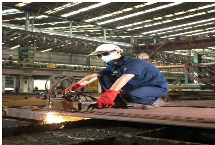
Gambar 4.11 Proses Flame Cutting
