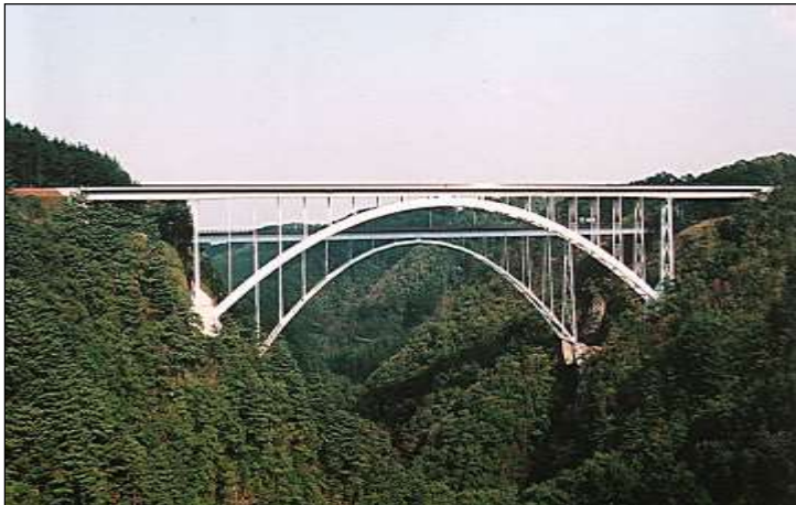
Gambar 2. 1 Jembatan Tipe Deck Arch
