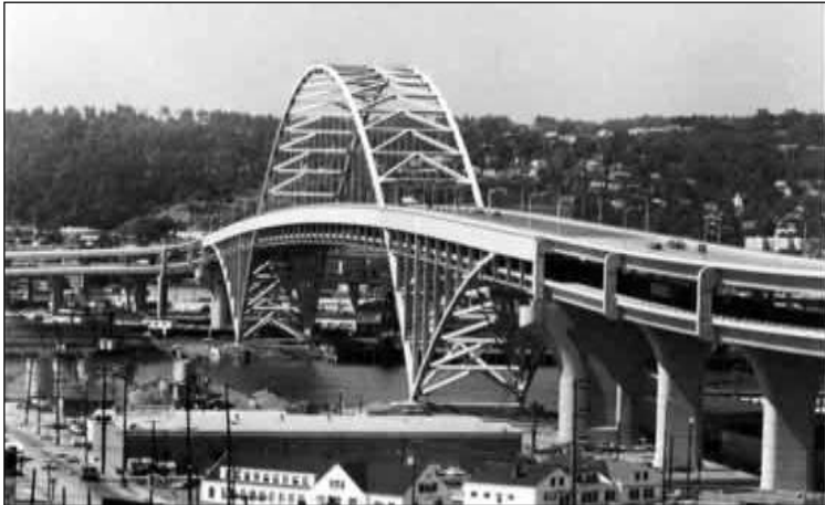
Gambar 2. 3 Tipe Jembatan A Half – Through Arch
