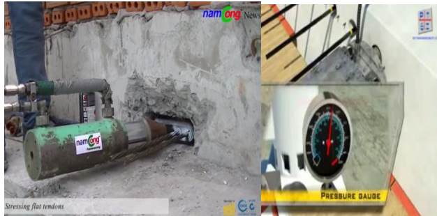
Gambar 4.135. Stressing Tendon Slab
