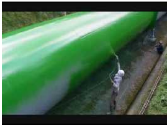
Gambar 2.16 Proses Pengecatan Pipa
