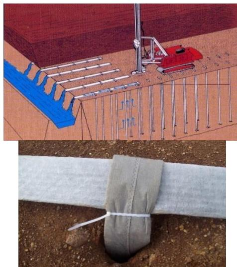
**Gambar 2.15** Pemasangan Prefabricated Horizontal Drain
