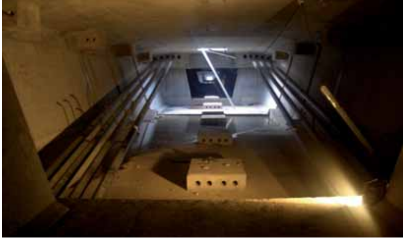
East Tsing Yi Viaduct, Hong Kong - 2009
