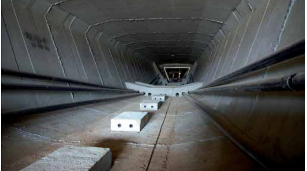
Gautrain Rapid Rail Link, South Africa - 2009
