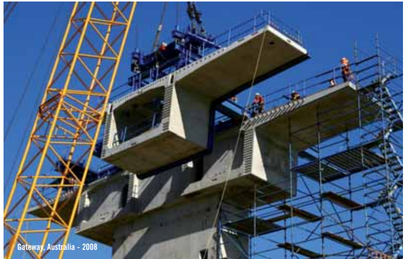
VSL executes all works using its own staff and equipment.
