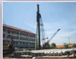
Piles Foundation for Building
