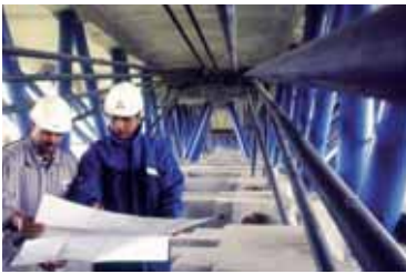
Boulonnais Viaduct, France - 1996
