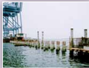
Piles for Marine Structure
