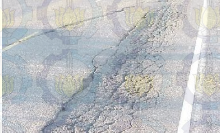
Gambar 2. 11 Alur (Rutting)
