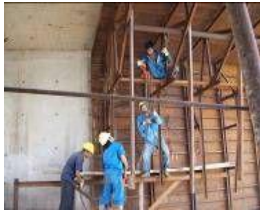
Gambar 4. 62 Outer Formwork
