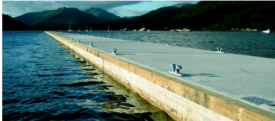
Gambar 4.1 Pontoon Floating Breakwater
